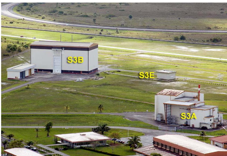
Figure 6.2.2.2.b – S3 area overview
